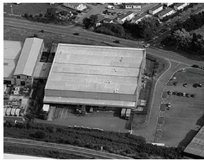
Early Felixstowe warehouse
