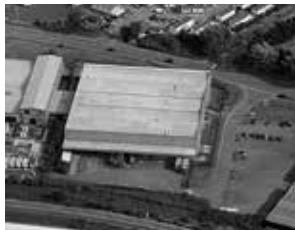
Early Felixstowe warehouse
